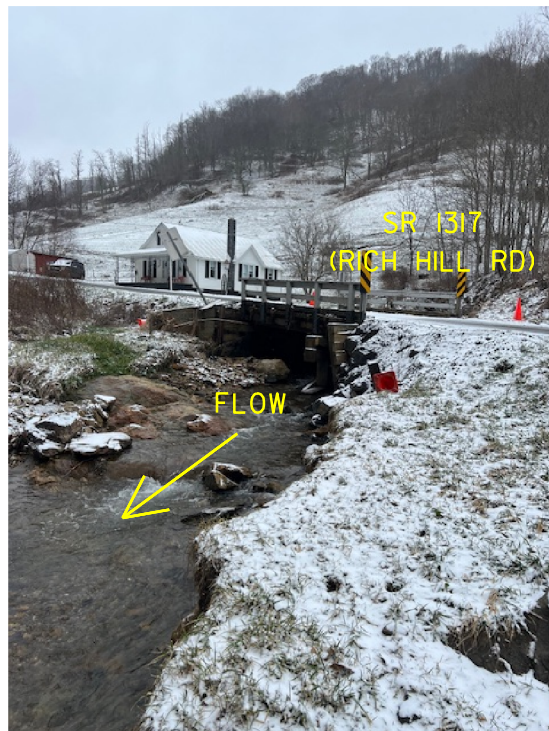
PHOTO #2: VIEW FACING NORTH DOWNSTREAM OF BRIDGE NO. 262.
